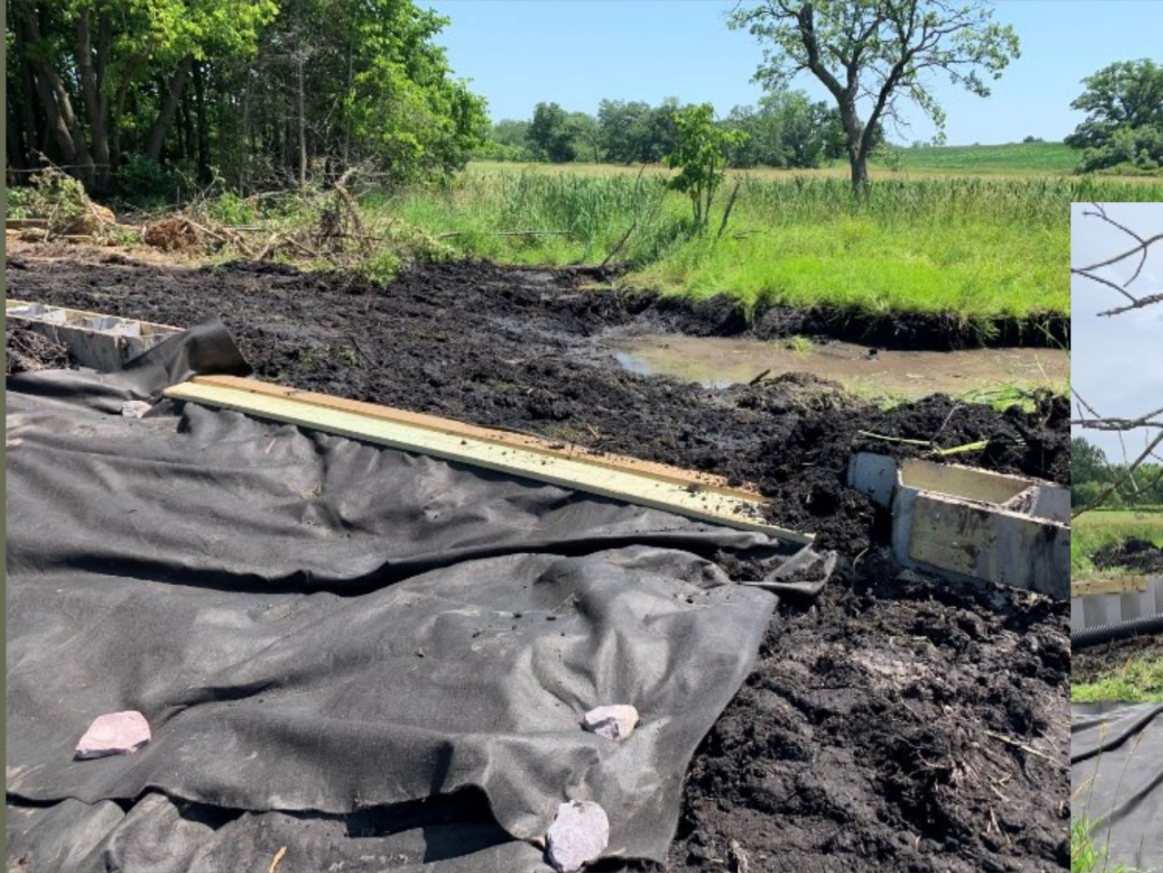
Fabric and stone install on spillway
