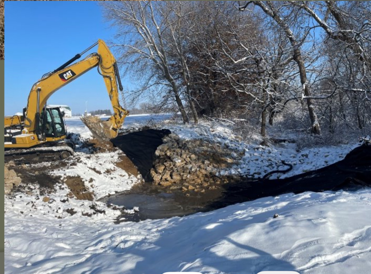
Installing fabric and rock
