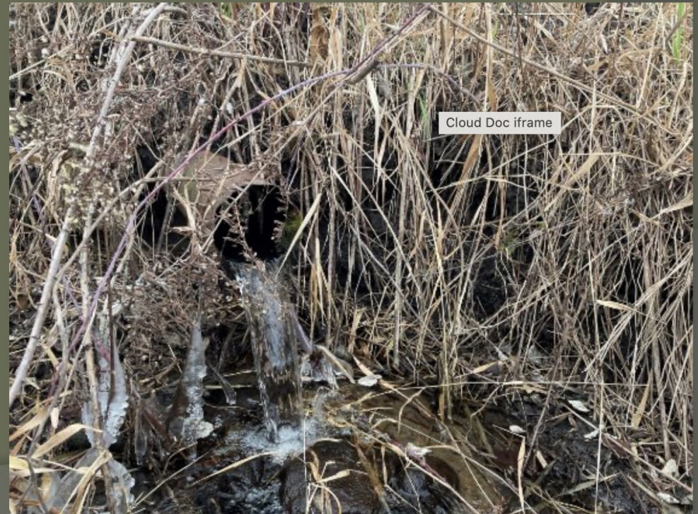
Finding Drain Tile
