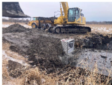
Installation of WCS
